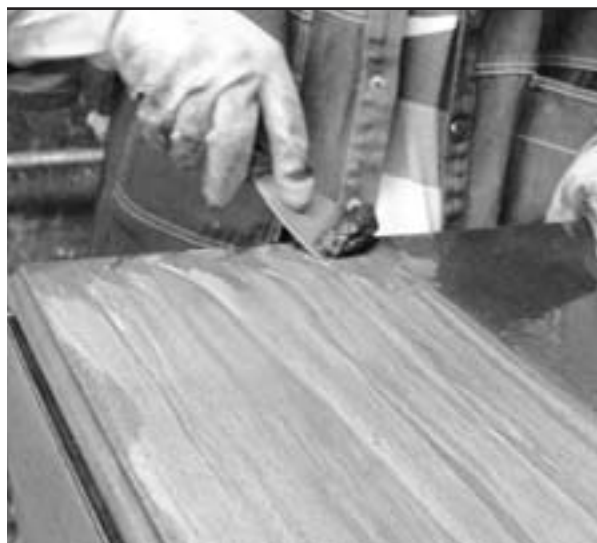
Apply paint stripper to small, workable areas.
