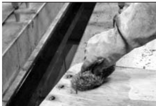
Wipe the stripped surface with a damp steel wool pad instead of hosing it down.
