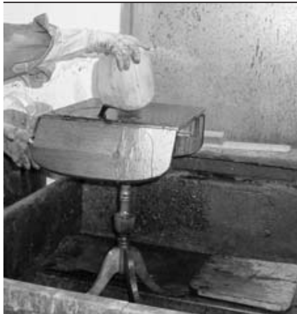
Capture and reuse paint stripper, if possible.
